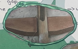
badly measured joint.
